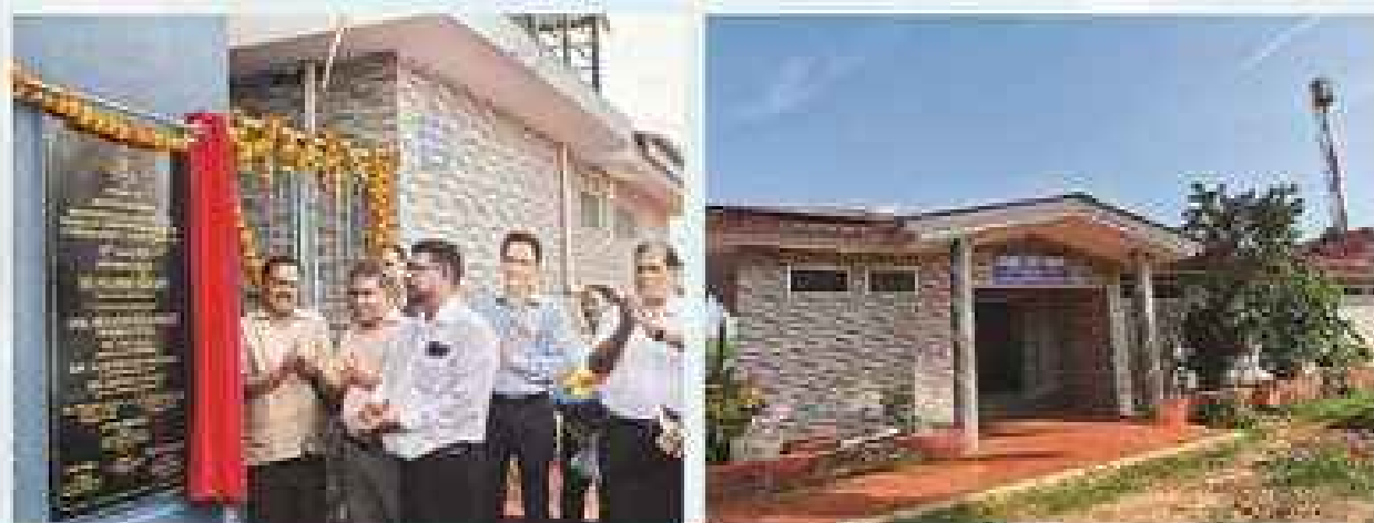
Newly constructed 50-seater Sulabh Shauchalaya Complex including Bathroom at cutbona Jetty
