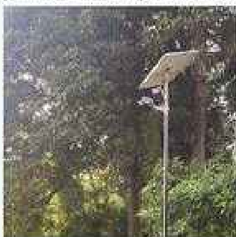
Solar Light panel installed at Nauxim
