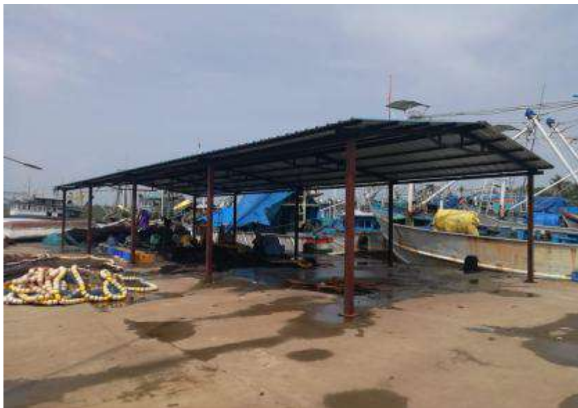
New Auction Shed at Cutbona Jetty
