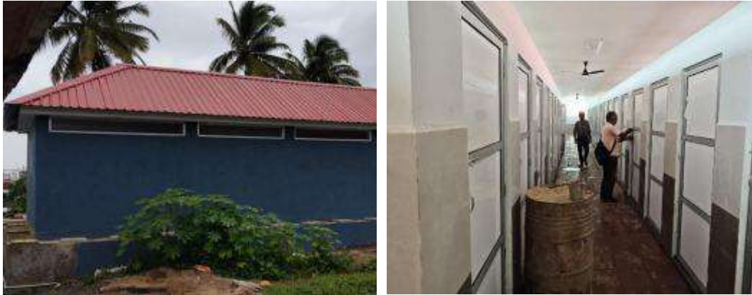
Under construction 50-seater Sulabh Sauchalay complex, at Cutbona Jetty
